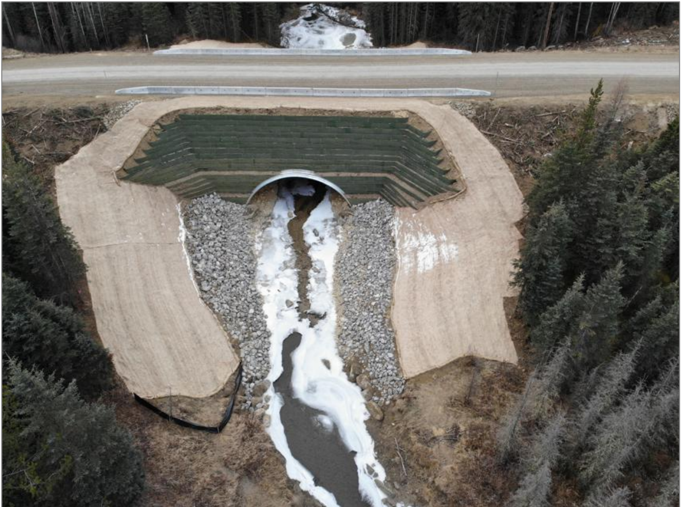
Figure 5. A Clear-span arch culvert is used to mitigate impacts to the aquatic critical habitat.
