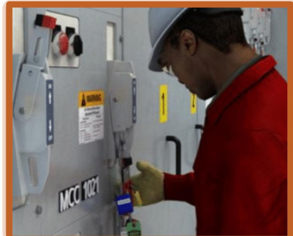
Lockout is a High Risk task. By providing lock out verification, another trained and competent worker double checks lockouts, which minimizes the risk of making a mistake in the Lockout process.
