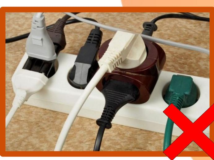
Don't plug another electrical device or an extension cord into the same outlet as a heater, it can cause overheating.
