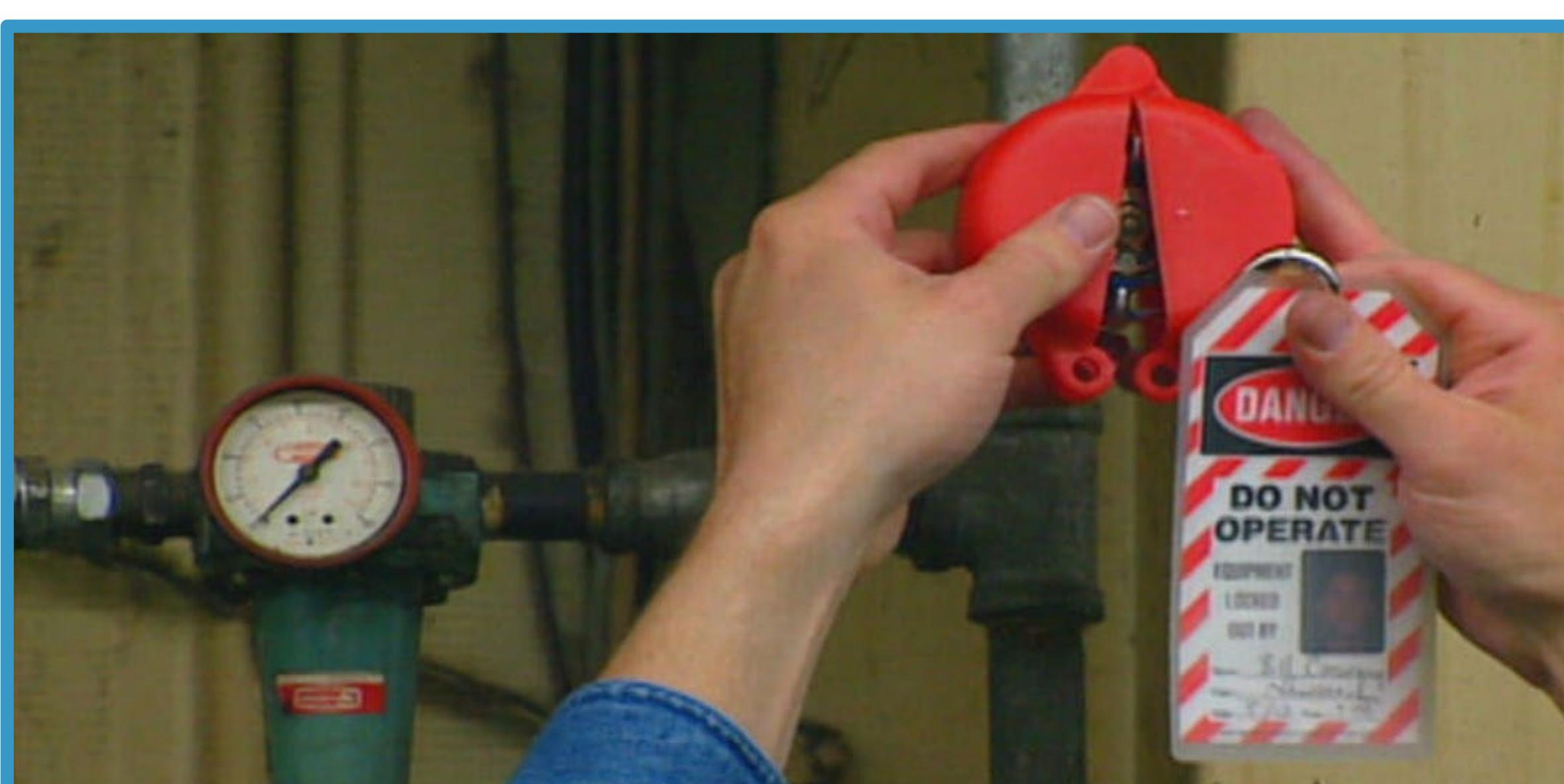
Live work is considered a last resort when performing work on energized equipment, and requires training and a permit. If possible, energized equipment should be locked out before work is done.
