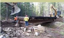
Temporary bridge being removed during class 4 road reclamation
