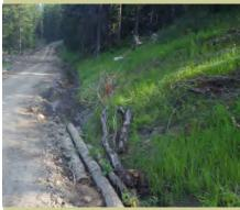
Cut-slope stabilization measures used by a disposition holder to prevent erosion (hydroseeding, debris placement, native vegetation staking)
