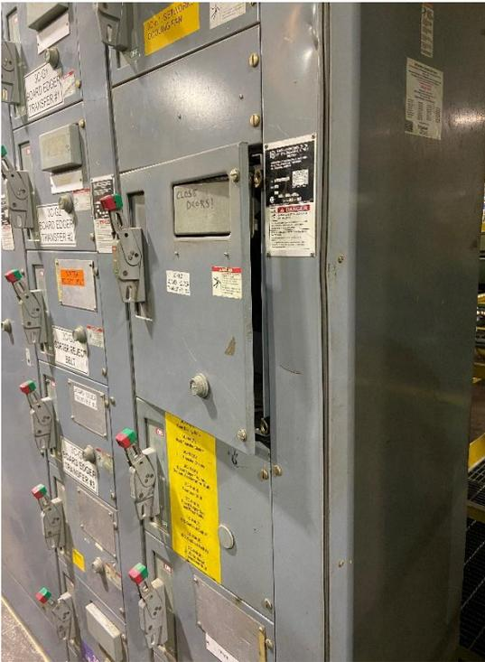
MCC doors that are left open decrease the safety design of the can/MCC in the event of an arc flash. Notify the shift electrician immediately.
